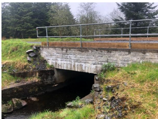
Plate 4-10 Bridge within the Wind Farm Site approximately 1.3 km west of turbine T10, showing modern concrete construction.
