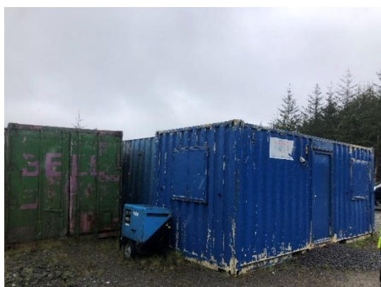
Plate 4-12 Prefabricated buildings, showing sealed construction and absence of bat roosting features.
