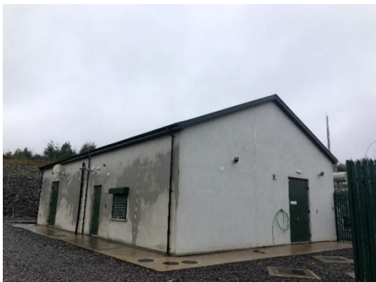
Plate 4-8 Substation Building 1 showing solid construction and sealed exterior.
