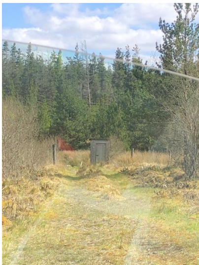
Plate 4-7 Small concrete shed with no gaps, cavities or other features suitable for bat access or roosting and assessed as Negligible roosting potential
