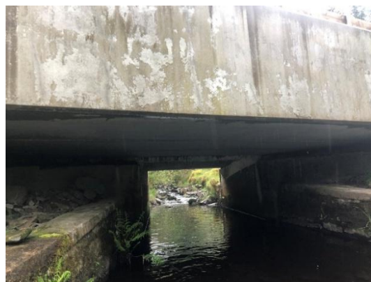
Plate 4-11 Underside view of bridge showing absence of features suitable for bat roosting.
